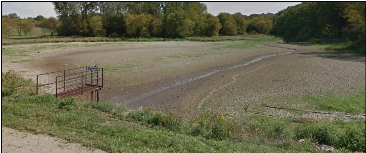
Figure 6. Sediment Basin Located on a Large Lake in Rural NW Illinois - View from Dam
