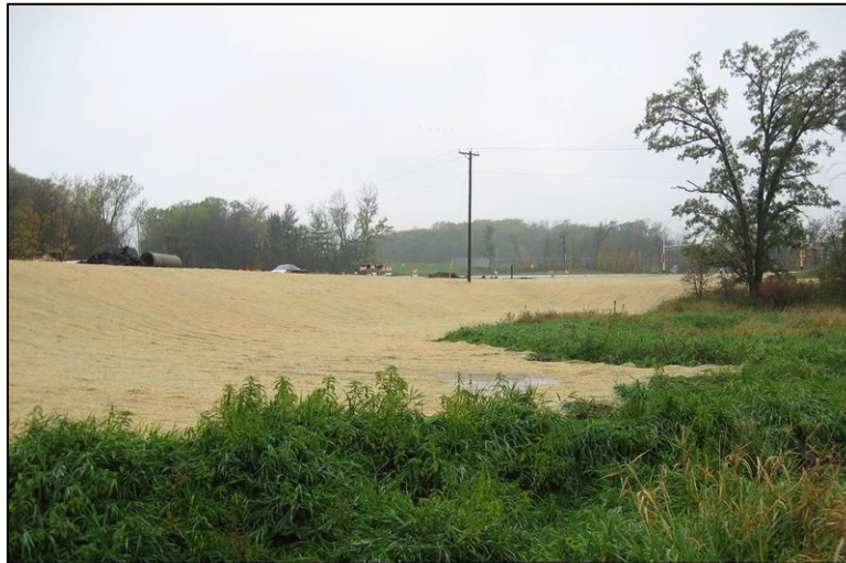
Figure 3. Example of properly applied mulch at a construction site ( https://stormwater.pca.state.mn.us/index.php?title=File:Mulch_stabilized_slope_2.jpg )
